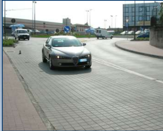
Roundabout – Palazzolo sull’Oglio (BS)
