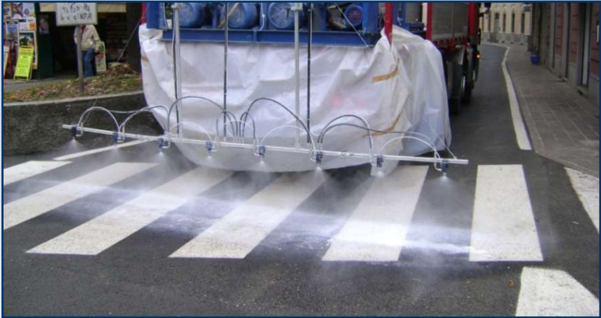
Bituminous pavement sprayed with photocalytic emulsions
