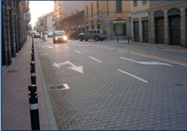
Photocalytic cement blocks pavements
